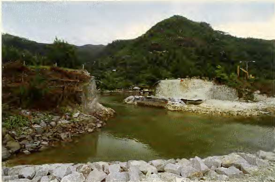
Plate 3. Road bridge washout from seaward drainage of tsunami waters from coastal lagoon, west coast of Mahé.
